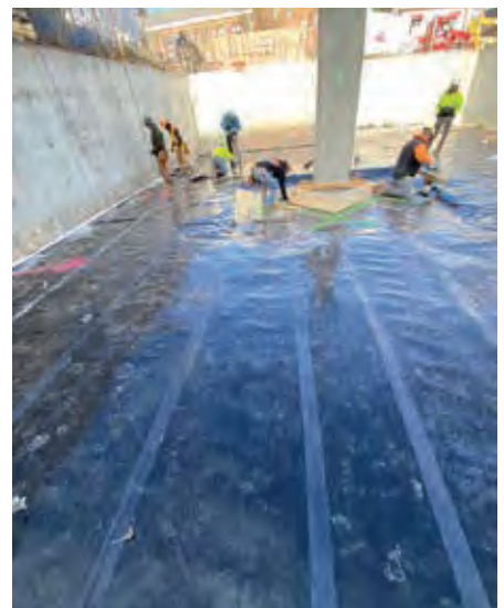
▲ Avenue E Underslab Waterproofing - Hoboken, NJ
